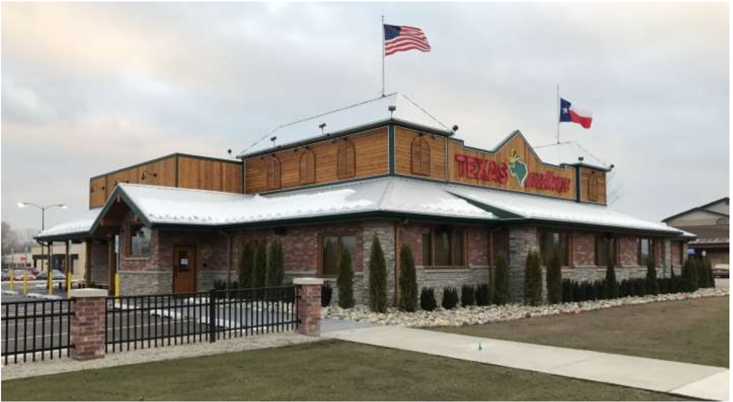
Texas Roadhouse opened in December at 2177 S. Mission in front of JC Penney.
